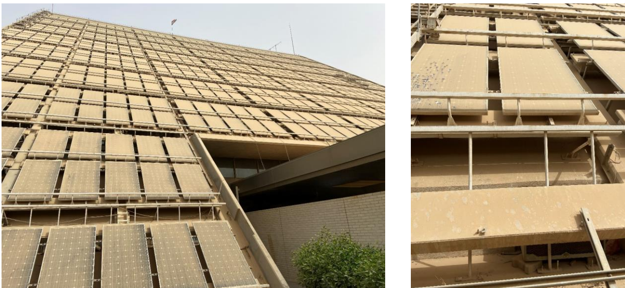
Figure (3): The REERC PV system a day after the May 17, 2022 dust storm.
