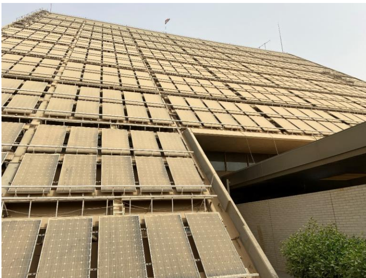
Figure (3): The REERC PV system a day after the May 17, 2022 dust storm.
