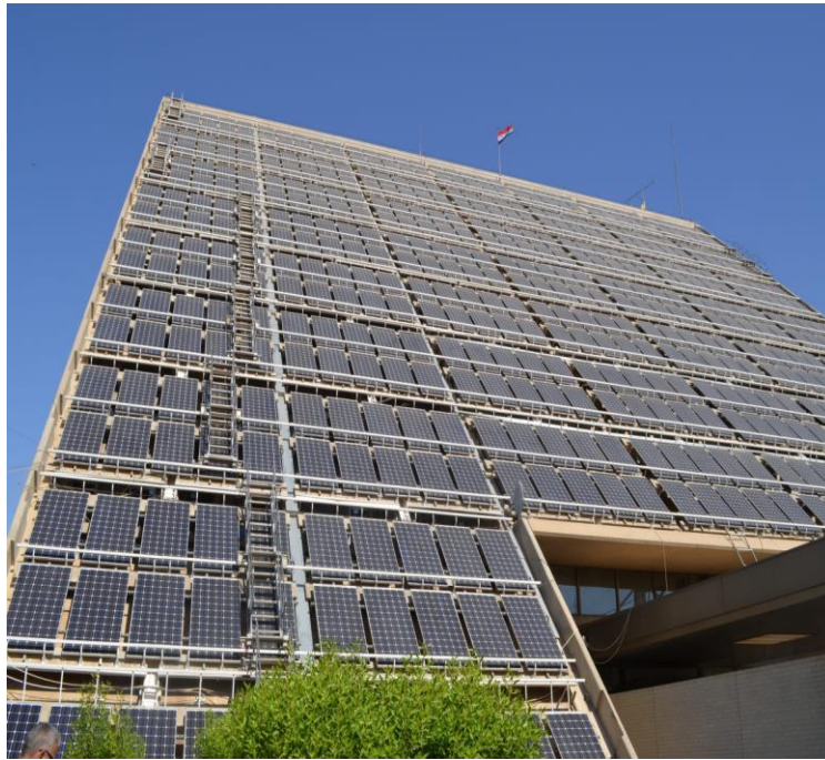
Figure (2): The 135kW REERC PV system.
